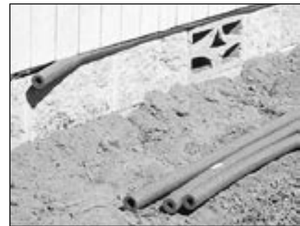
Tip: Plug that 1-inch clearance with lengths of foam pipe insulation to ensure protection from rodents.
